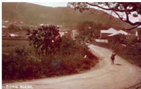
Lawrence Hargrave Drive in a time before traffic jams. Photo: Illawarra Images/Wollongong City Libraries
